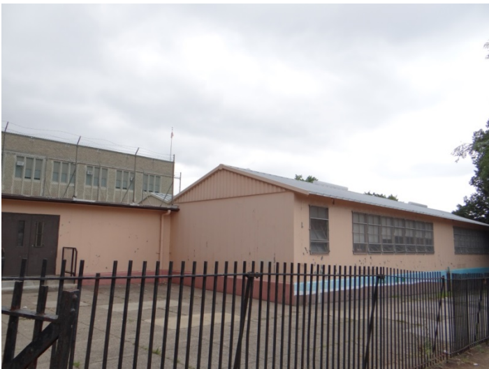
Photo 5: Looking N at portables addition at E side of school
