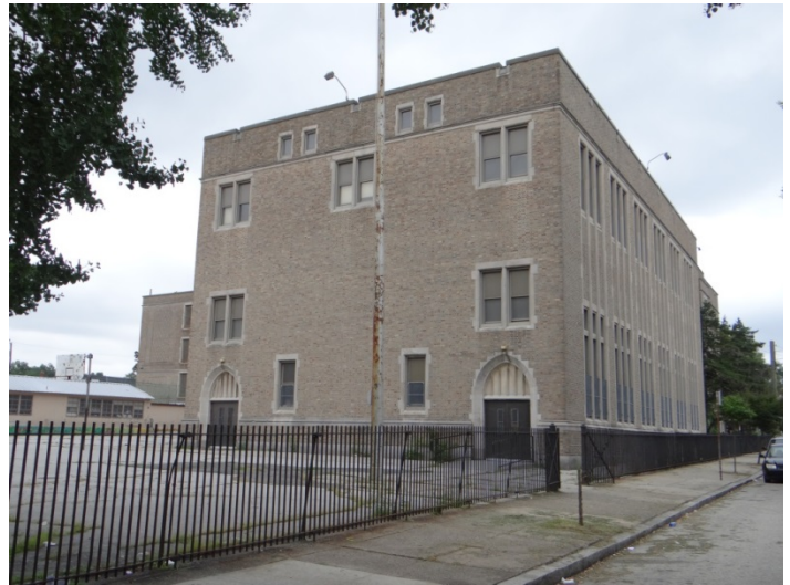
Photo 4: Looking S at NE end of addition
