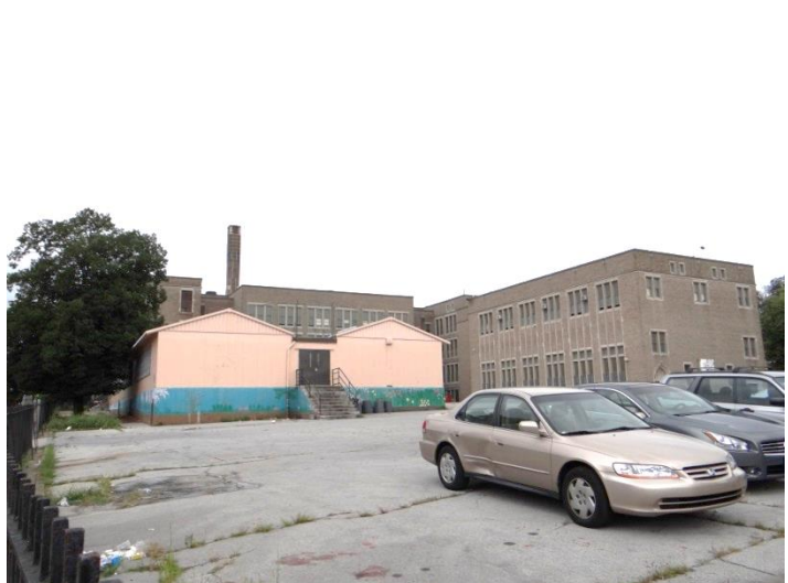
Photo 6: Looking W at rear (E) facade
