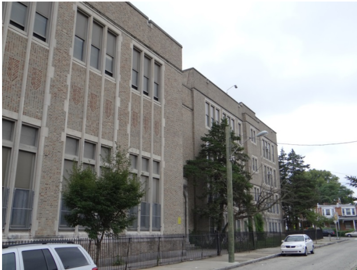
Photo 3: Looking S at NW façade, addition to left
