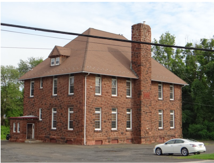
Photo 1: Looking N at main (SE, right) and SW (left) facades
