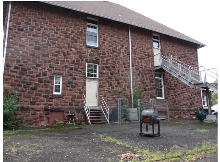
Photo 4: Looking SE at rear (NW) facade
