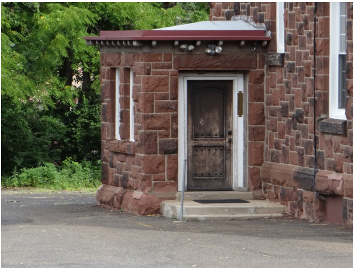
Photo 3: Looking W at entrance on SW facade
