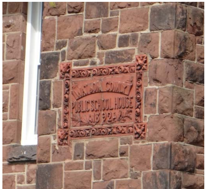
Photo 2: Detail, datestone, main (SE) facade
